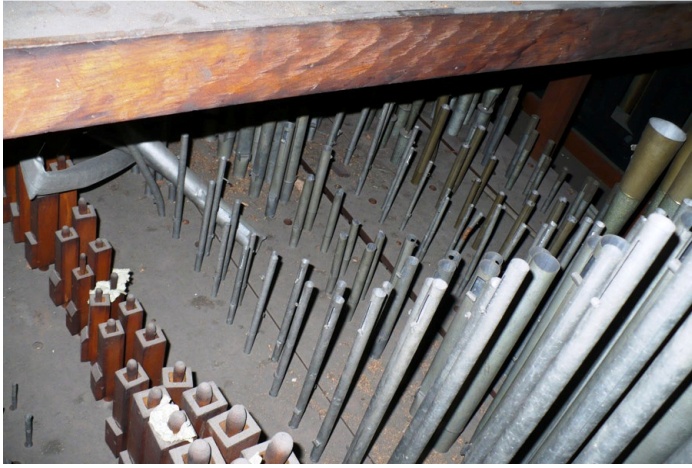
Pipework from overhead
