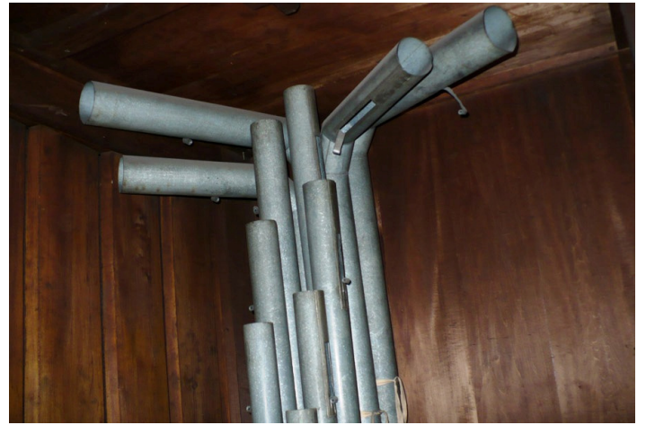
Choir pipework looking up
