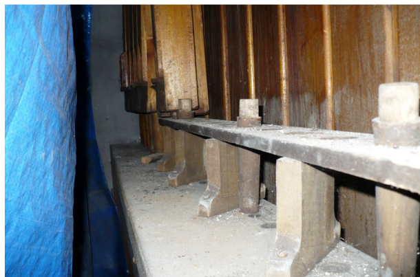
Missing Bourdon pedal pipes
